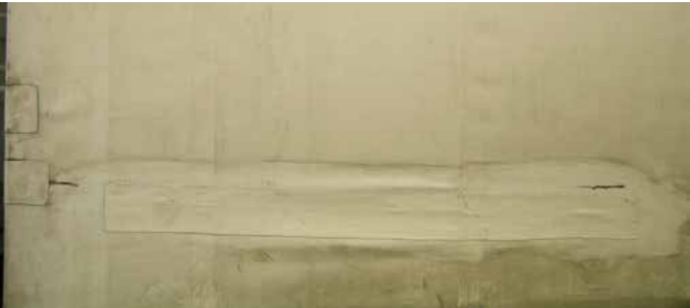
✓ Repair work carried out professionally on the tarpaulins
