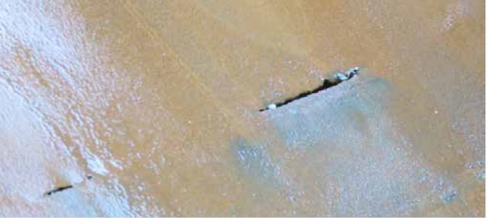
✗ Cracked tipper pan
