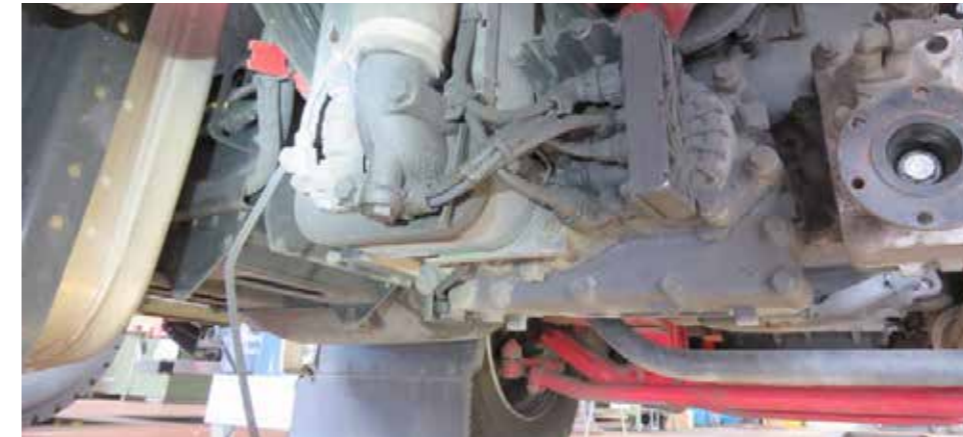
✓ Gearbox with slight oil moisture
